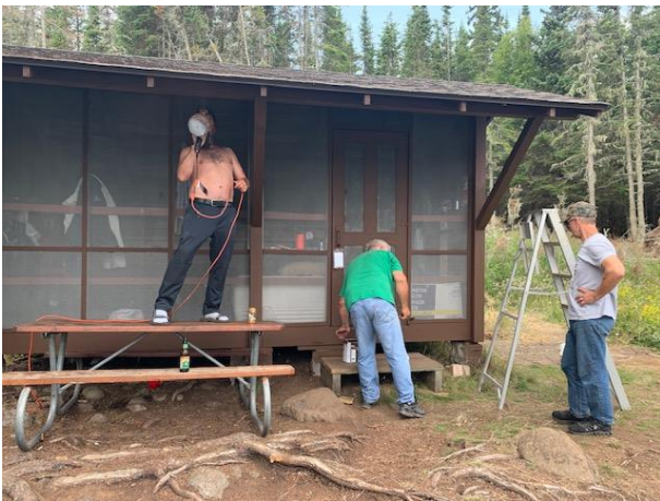
IRBA members finishing up painting the shelter.
